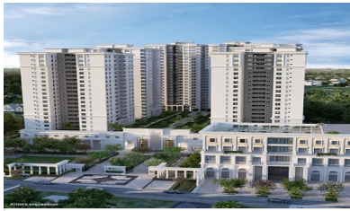
Sobha Neopolis Construction Status
